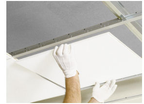
The individual tiles are easily demountable
